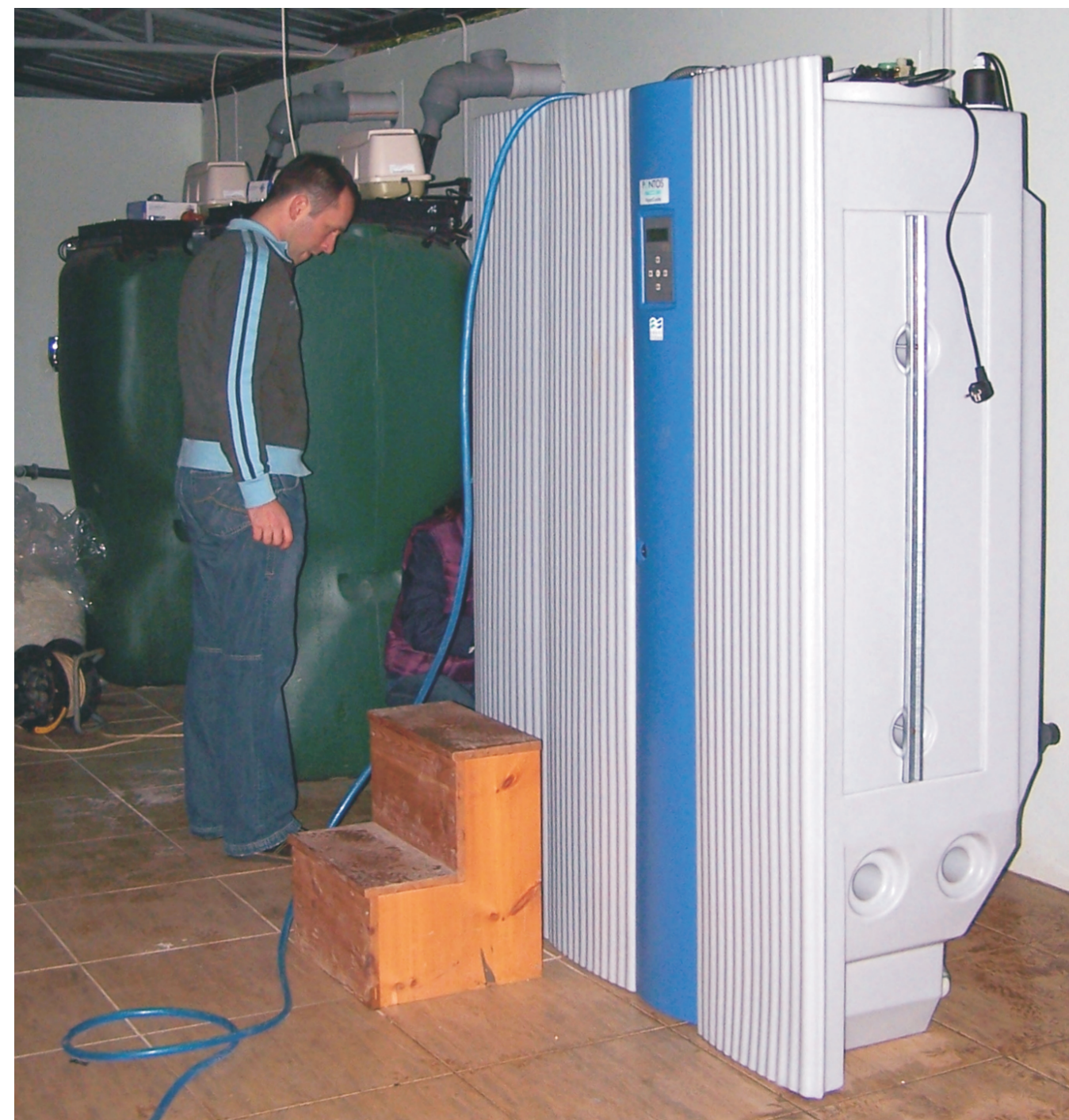
Introduction of new techniques - Inhouse SBR greywater treatment
