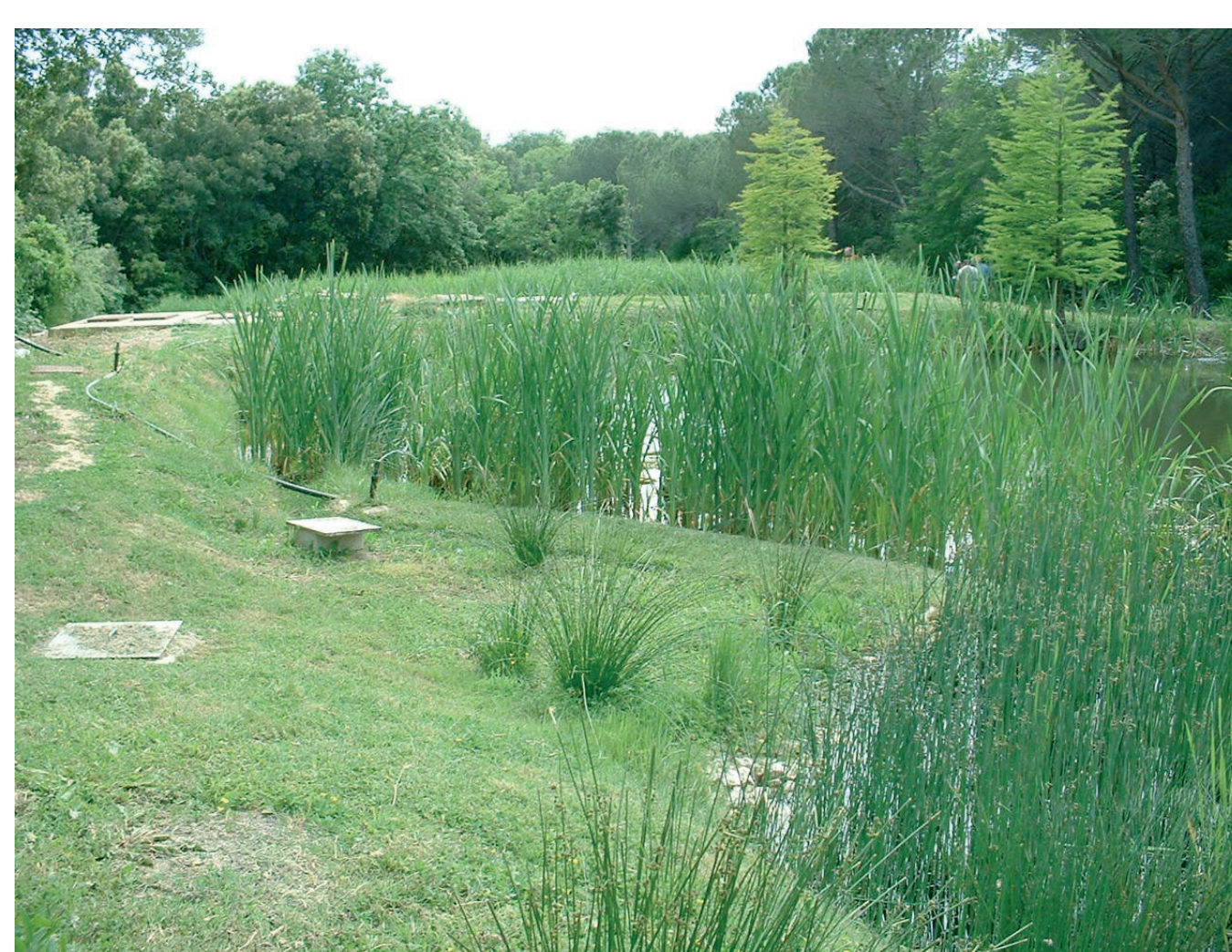
Appropriate techniques - Constructed wetland in Italy, a treatment with low energy and maintenance requirements
