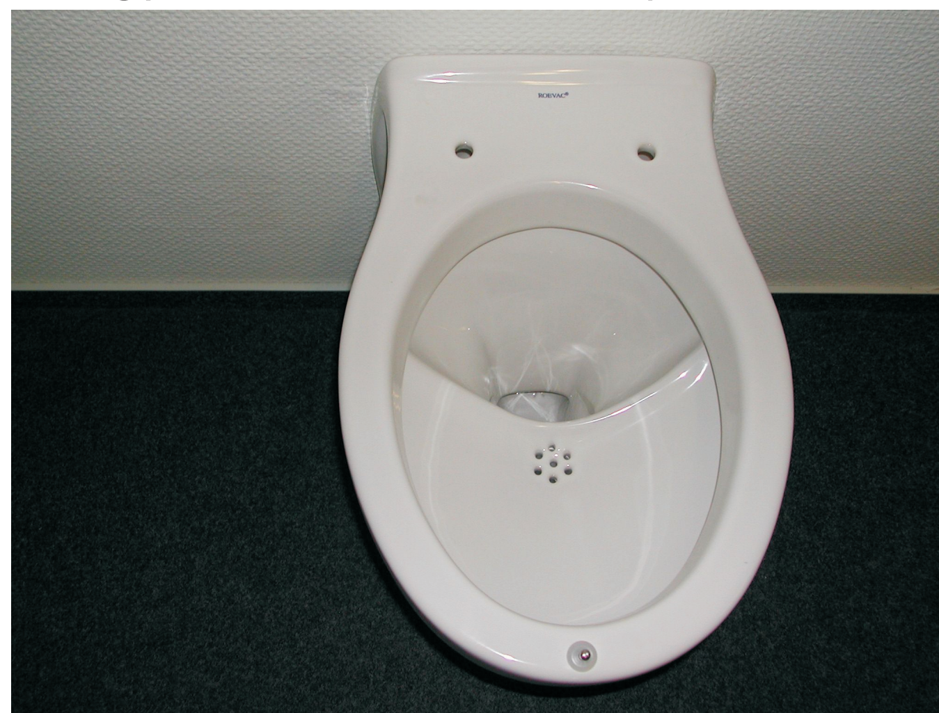
Integrated approach for reuse - urine separation toilet as example for a good practice
